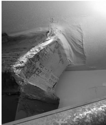
Fig. 9. Ductwork hole repaired.
