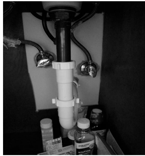
Fig. 8. Holes sealed under bathroom vanity.
